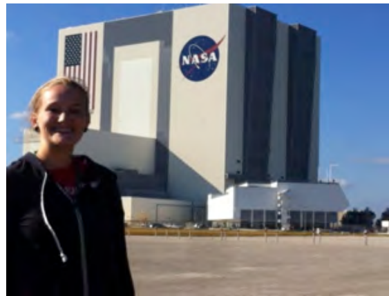
The Vehicle Assembly Building at KSC, the third largest building in the world by volume. Credit: Taylor Garber
